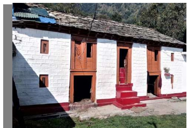
Fig-3: Traditional homestay in sarmoli village in the second Floors.
